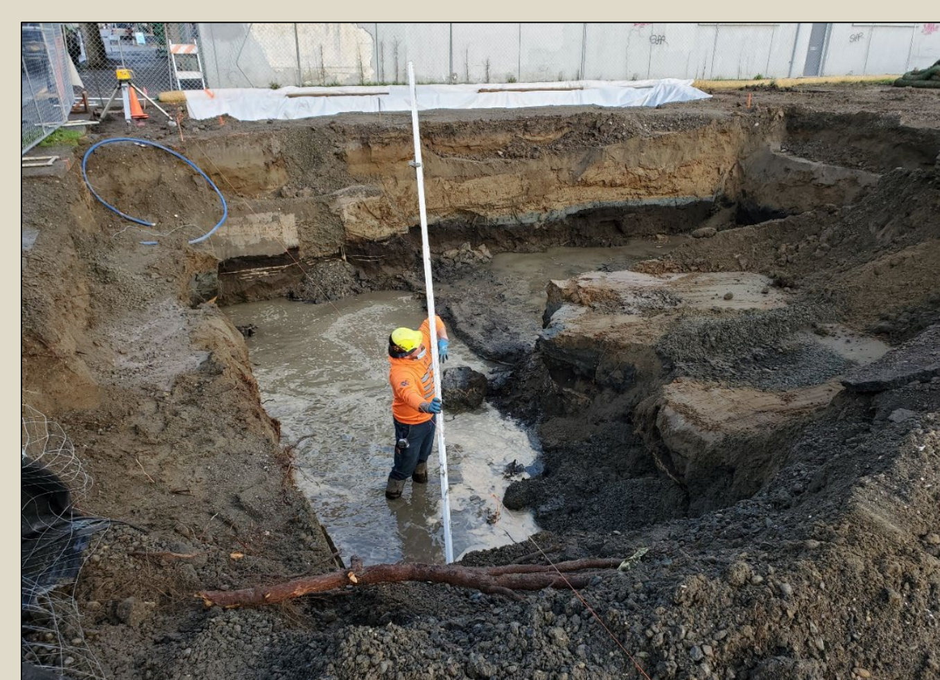
Figure 2. Foundation excavation in progress at 45TN519 at high tide, December 2020.
